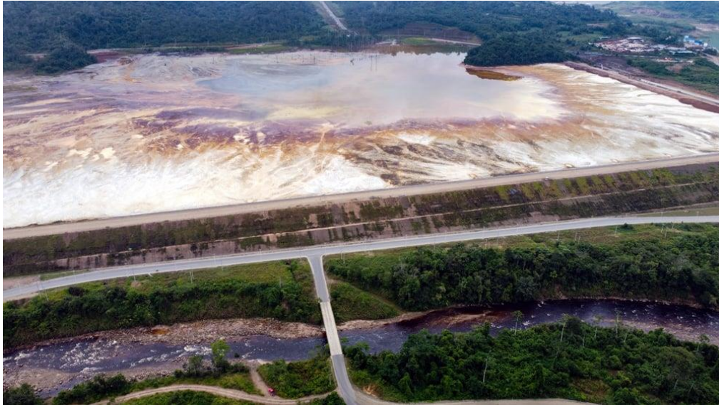
Figure 14: The Quimi tailing dam pond adjacent to the Quimi River
